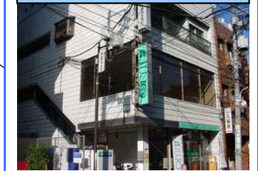
North Tokyo Office
